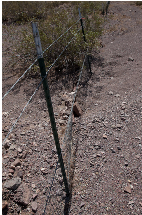
Typical tortoise fence installation
